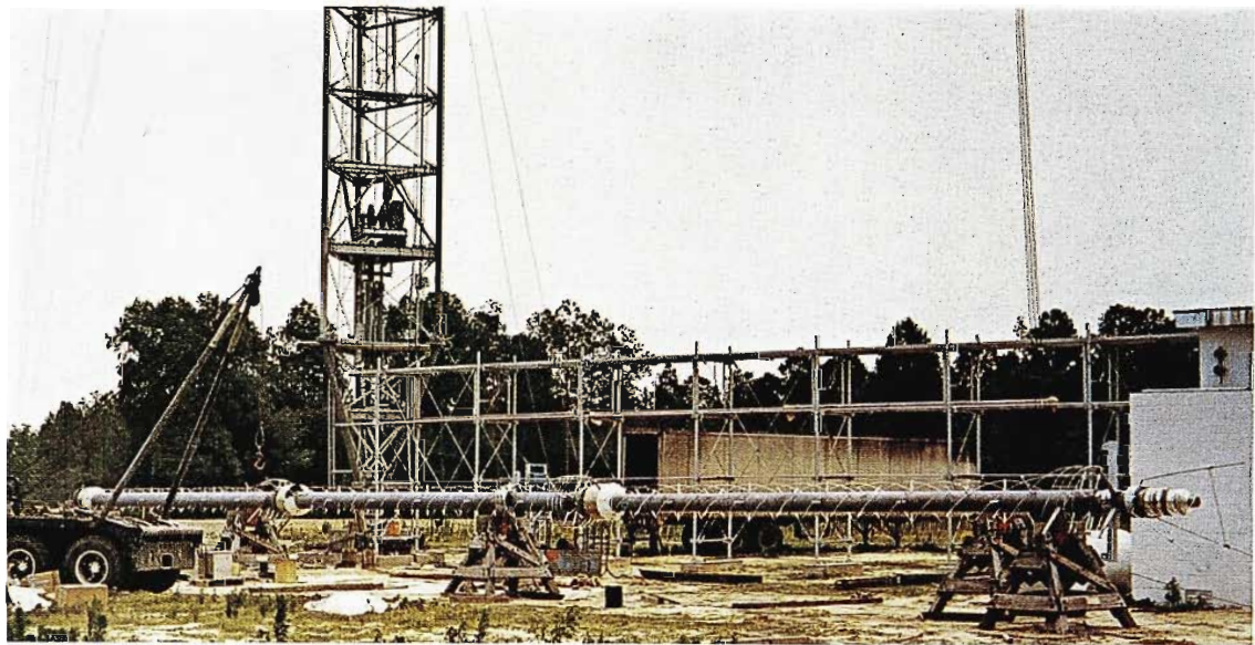
WBTW-TV's Tetracoil CP antenna was trucked from Gibbsboro, N.J. to the tower site at Dillon, S.C. in two pieces and was assembled on the ground.
