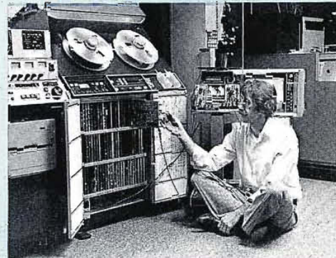
Greg Fox, Video Chief Engineer, maintains the high quality of equipment standards and operation. Here, a TR-600A quadruplex VTR is set-up to facility requirements.
